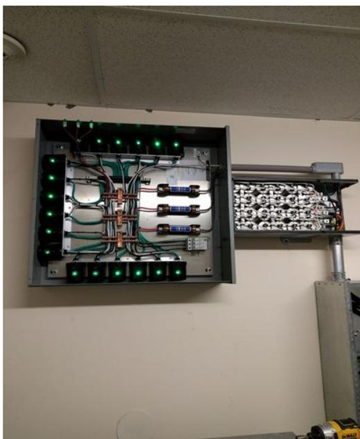
480 Volt / 100 KVAR unit opened to expose the heart of the unit, the metal oxide Varistors shown above
